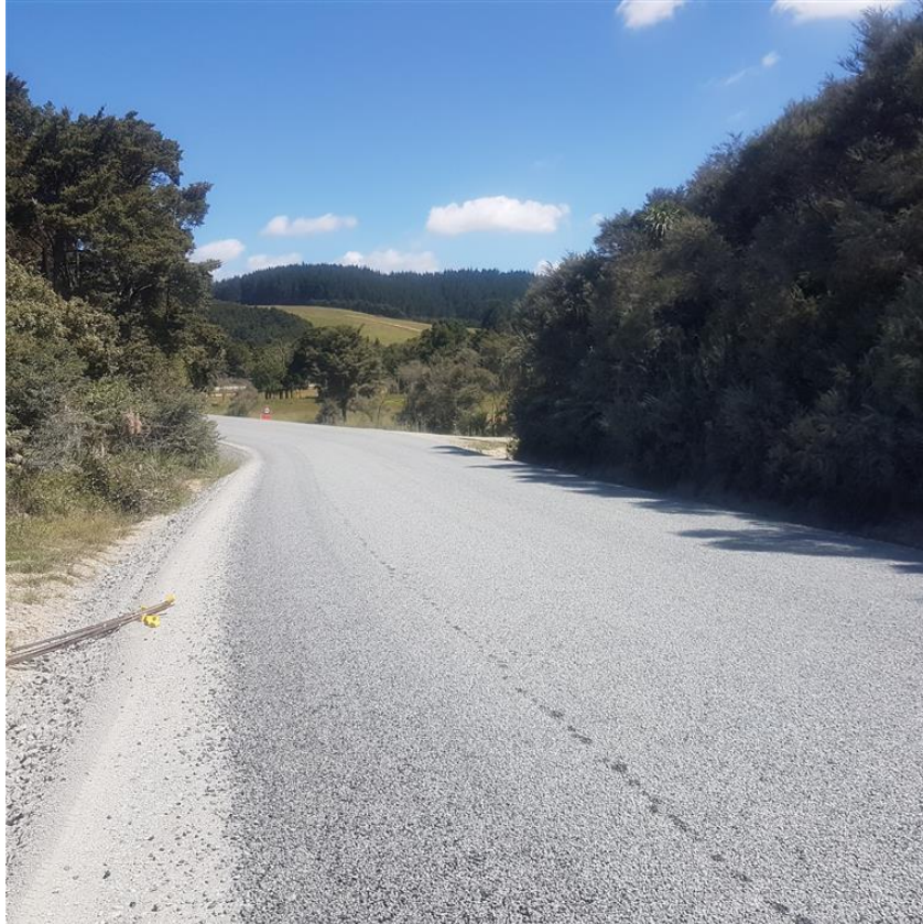
Wright Rd final section sealed
