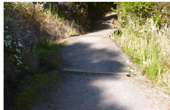
Raised box culverts along Boswell Track
