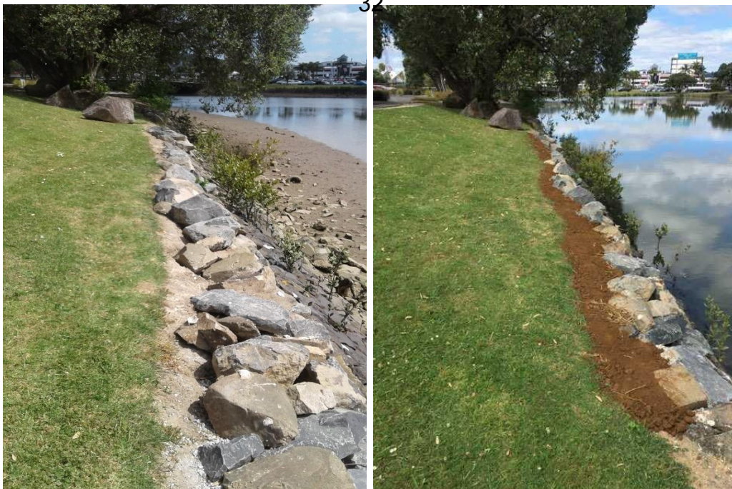
Aquatic centre seawall received dry stacked repairs and backfilling at several locations
