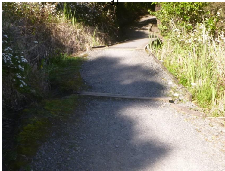
Raised box culverts along Boswell Track
