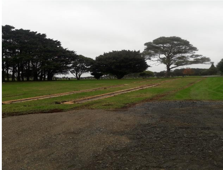
New burial plots under construction
