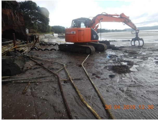
Illegal pipe seawall being removed
