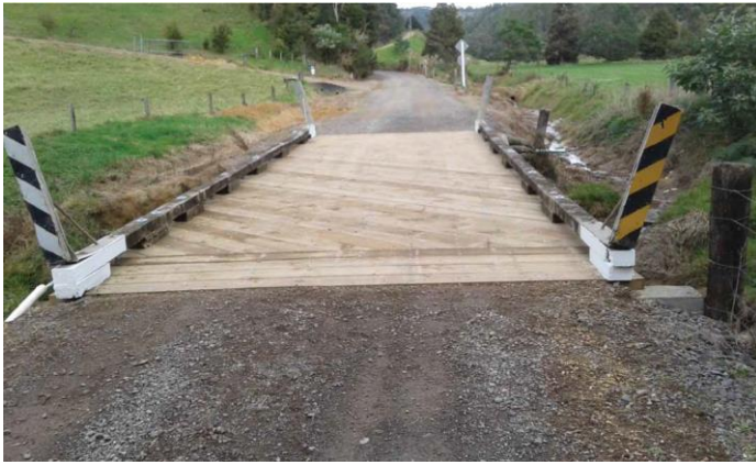
Jellick Rd Bridge Repair
