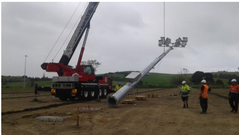
Lights being installed at Otaika Sports ground
