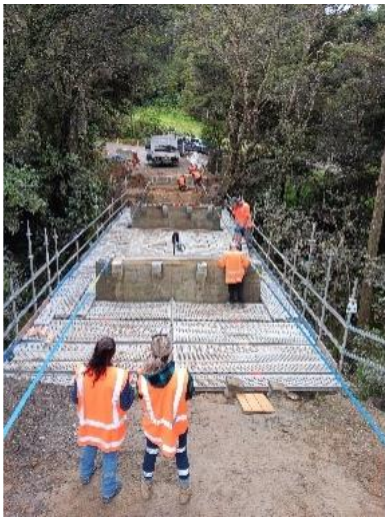
Waipu Caves Bridge - Old deck removed & piers prepared for new deck arrival
