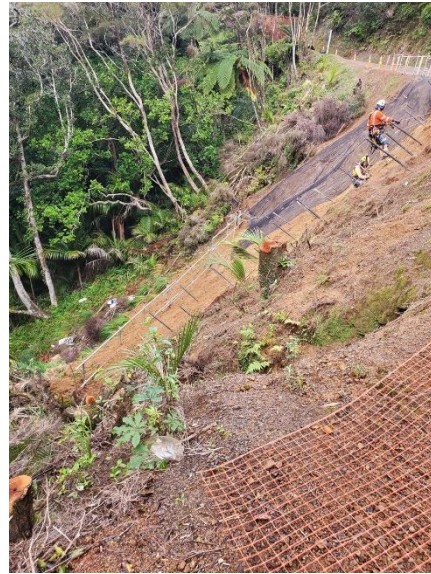
Emergency Works Phase 3 - WDC Slip Package 1 - Kaiikanui Rd – Installation of nett
