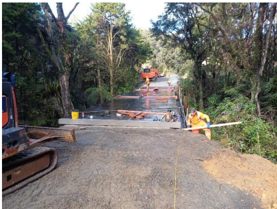
Waipu Caves Bridge - Old deck removed & piers prepared for new deck arrival
