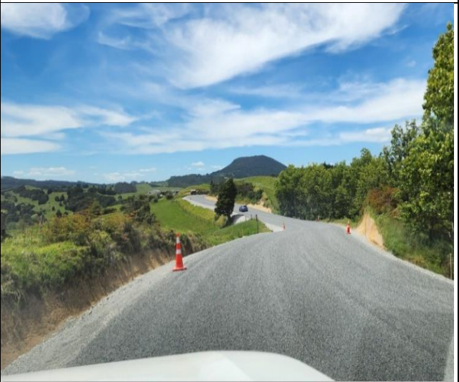
CON17086 Rd Mtce & Renewal Sth – Snooks Rd Rehab
