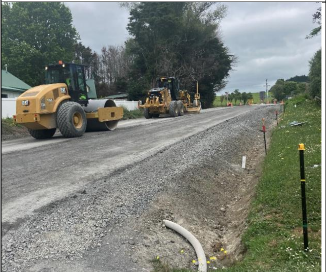
CON17085 Rd Mtce & Renewal Nth – Pipiwai Rd (ctrl) Rehab
