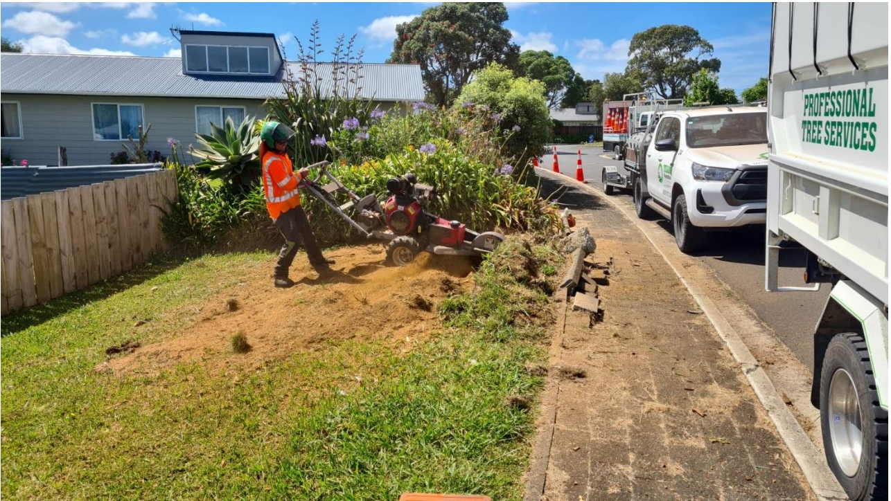
Stump removal and footpath repair – Aratiatia Place
