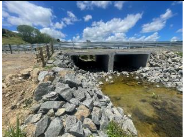
CON21039 - Mangapai Culvert
