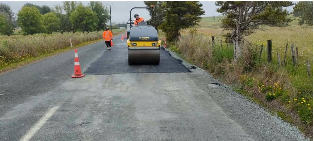
Sealed rutting repair – Springfield Road
