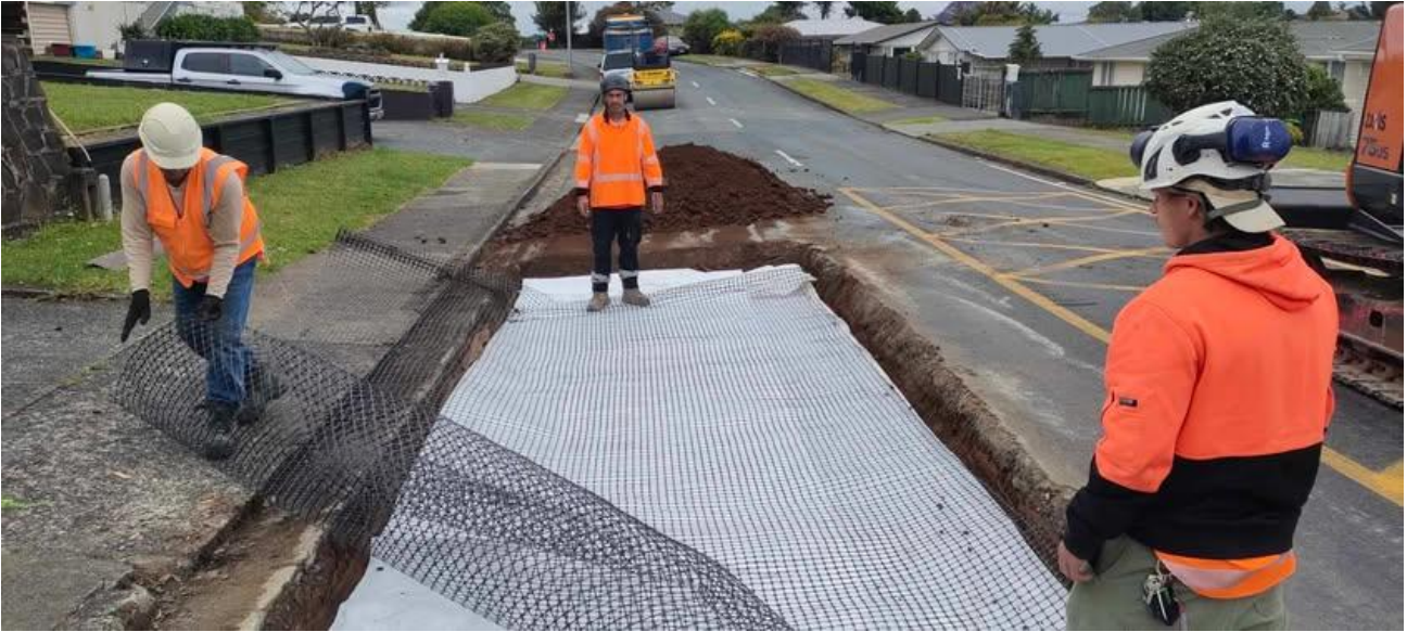
Digout repairs – Eden Terrace
