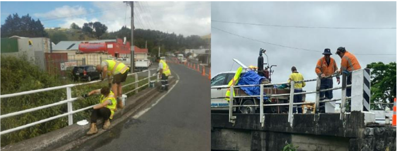
Bridge Rail Repairs – Hikurangi
