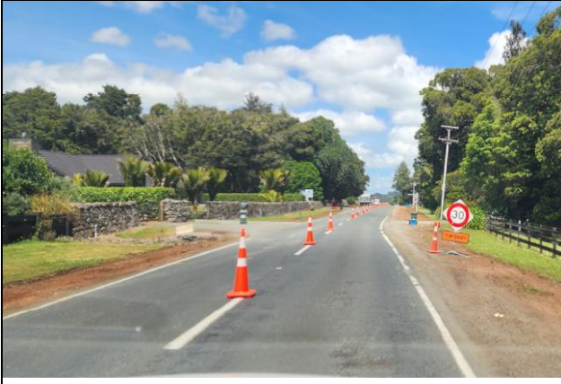
CON17086 Rd Mtce & Renewal Sth – Three Mile Bush Rd Rehab
