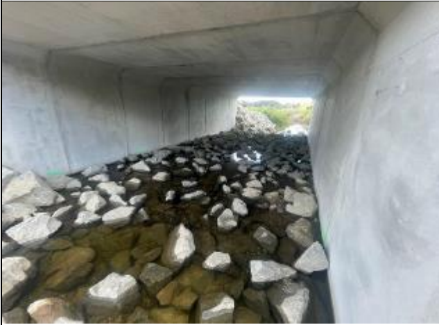
CON21039 - Mangapai Culvert
