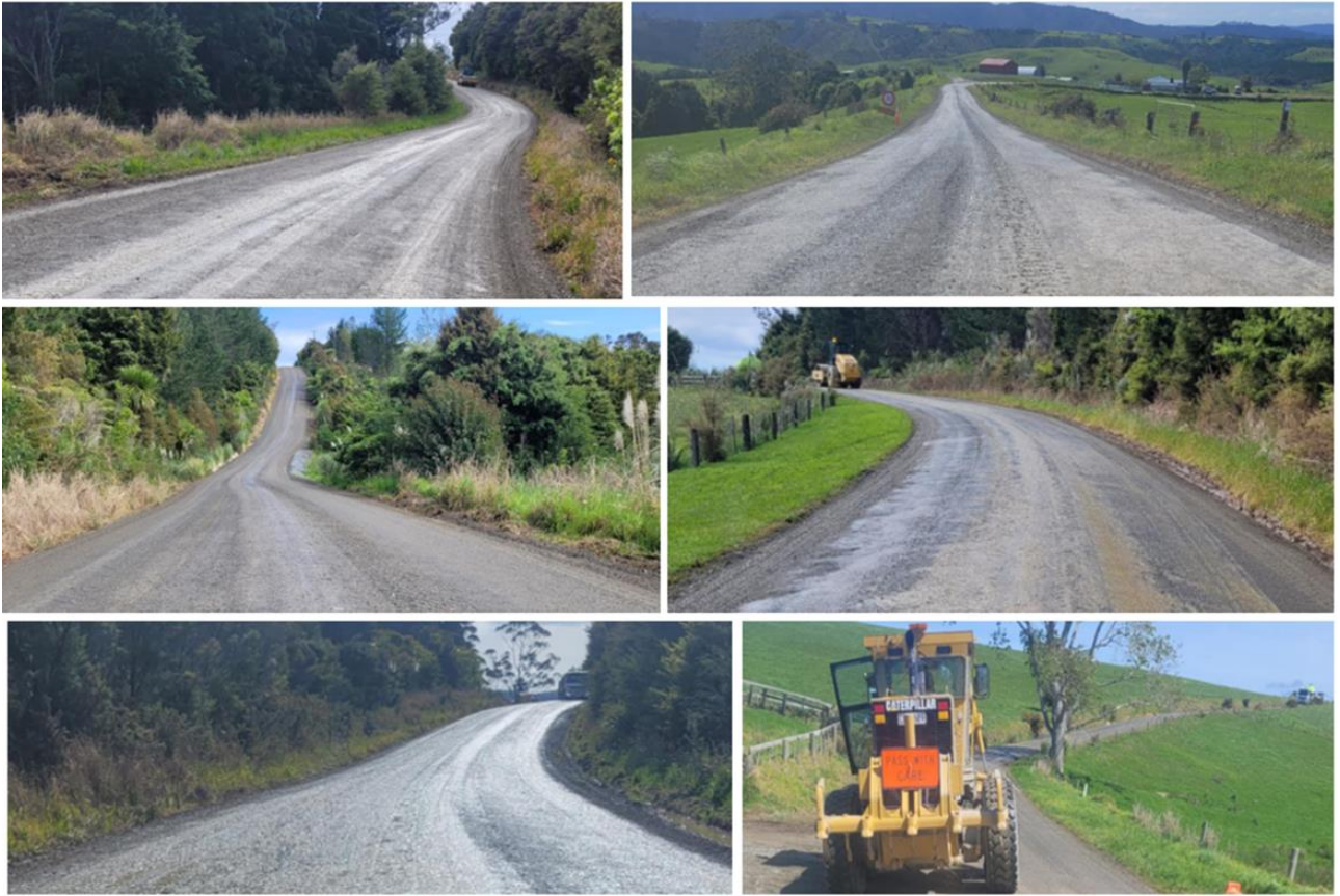
Unsealed Rehabilitation - Durham Road
