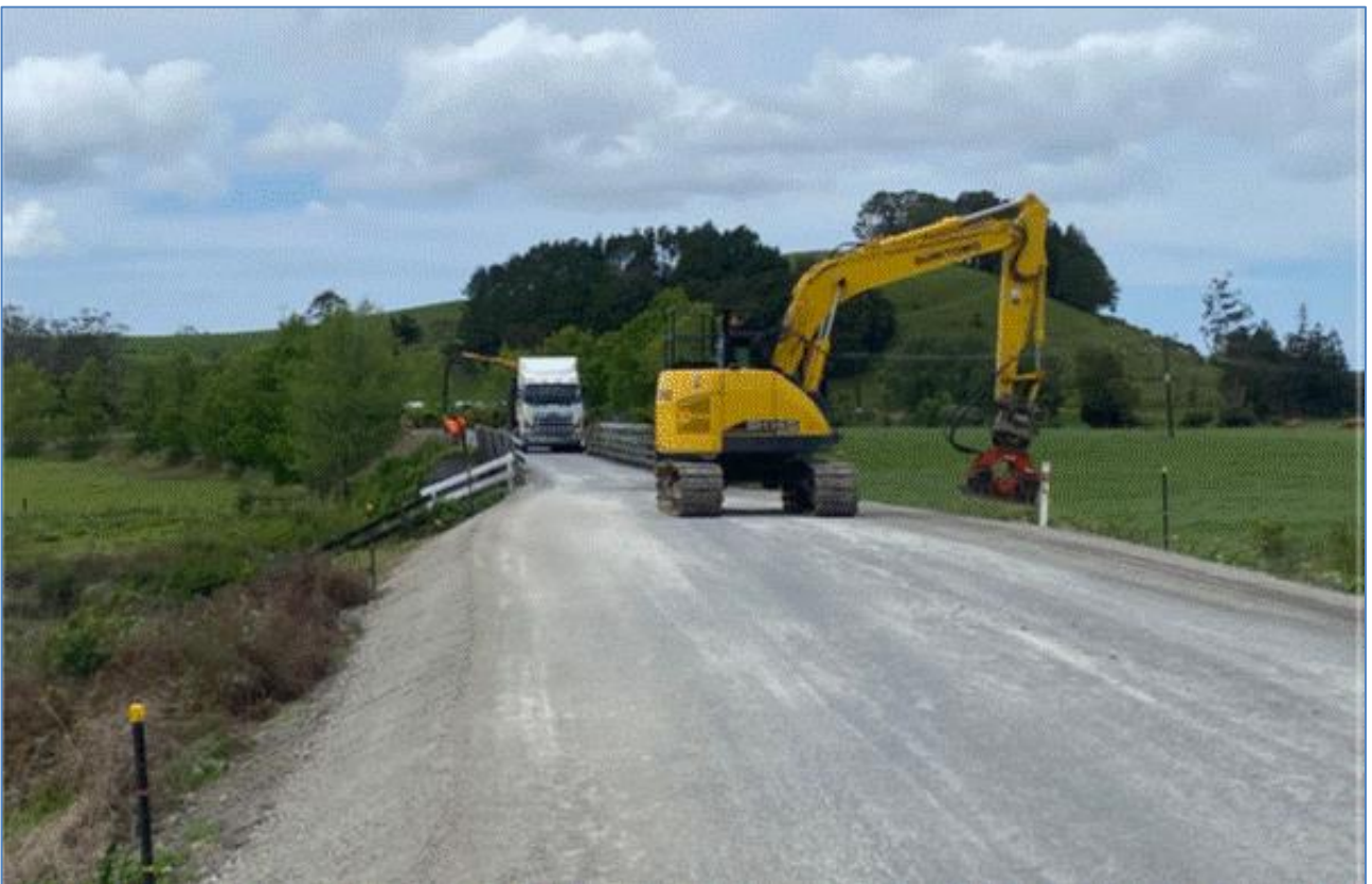
Sight Rail cleaning and painting – Whareora Road
