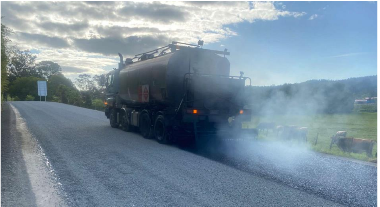
Rehab sealing – Russel Road
