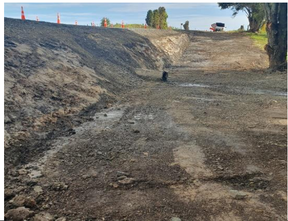
CON22091 SP1 Paparoa Road Slip Remediation – excavation for retaining structure
