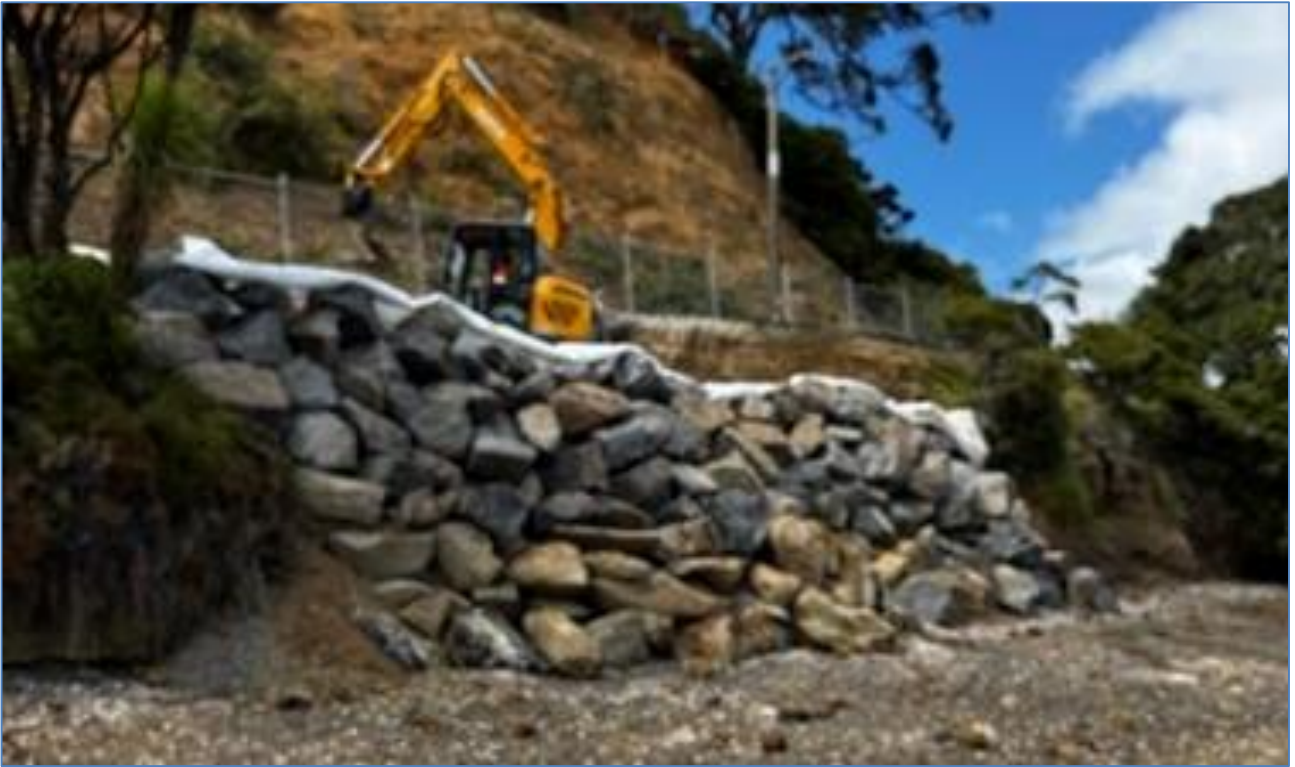
Underslip Repair - Whangaruru
