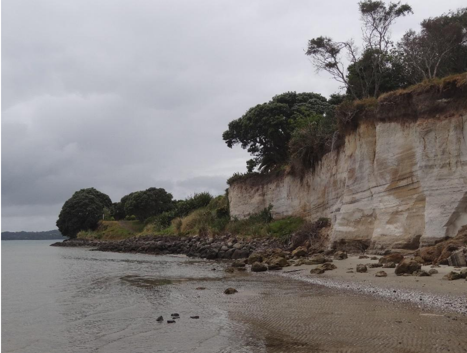
Photograph 2: Rock revetment to the north of the site showing stable angle of repose and vegetation establishment, in comparison to exposed cliff to the south. Source T+T 2014.
