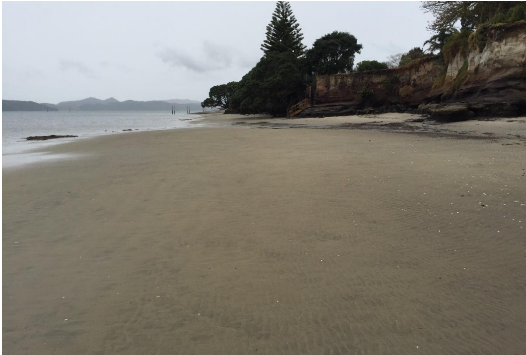
Figure 9: View of the beach looking north-east. Limited occurrences of Pleistocene shallow marine sediments can be seen exposed on the beach as extremely weak rock.
