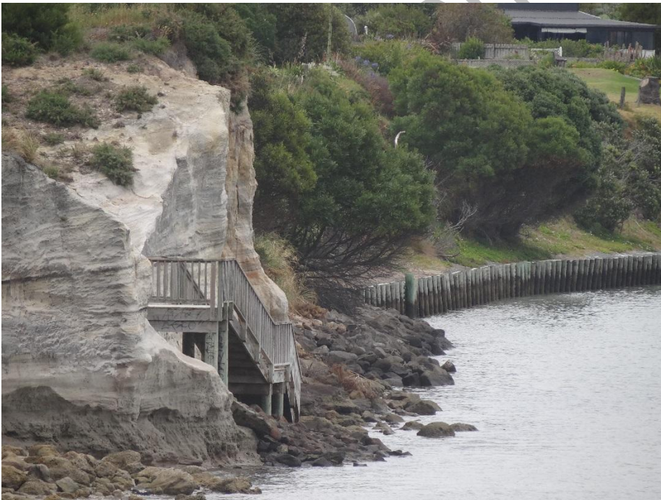
Photograph 3: Rock revetment and timber seawall to the south of the site. The slope is gradually flattening above the revetment. Source T+T 2014.
