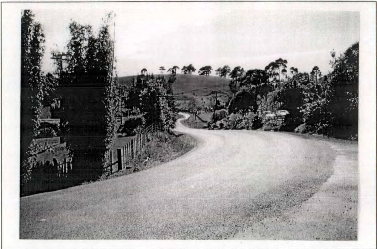
Photo 2 Looking East from the main entrance.
