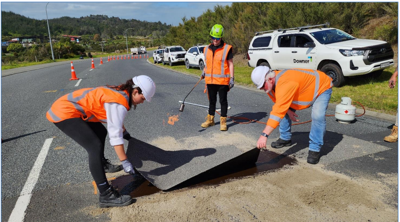
Downer BRP Patch Side-by-side trial – Kotata Rise
