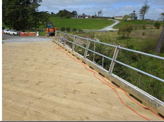
CON21086 – Thompson Road Bridge Upgrades
