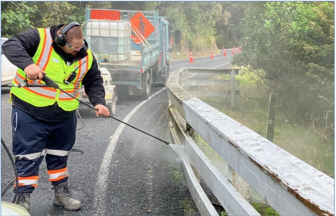
Sight Rail cleaning and painting – Whareora Road
