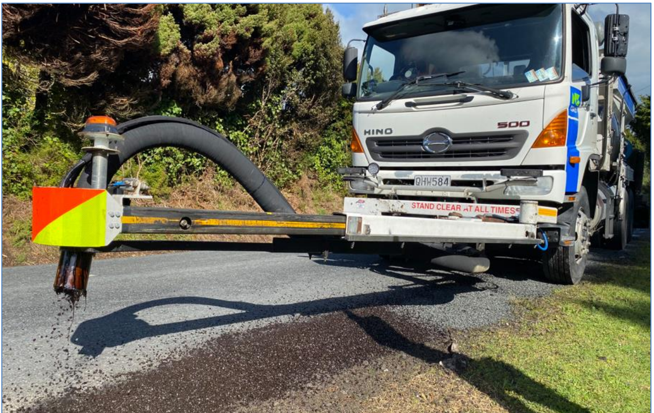
FH Jet Patching Unit repairing Edgebreak – Millington Road
