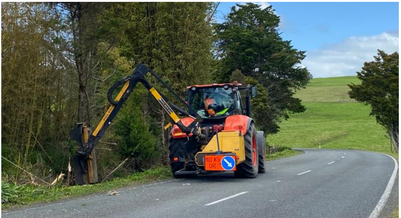
Improving Sight Lines – Pipiwai Rd
