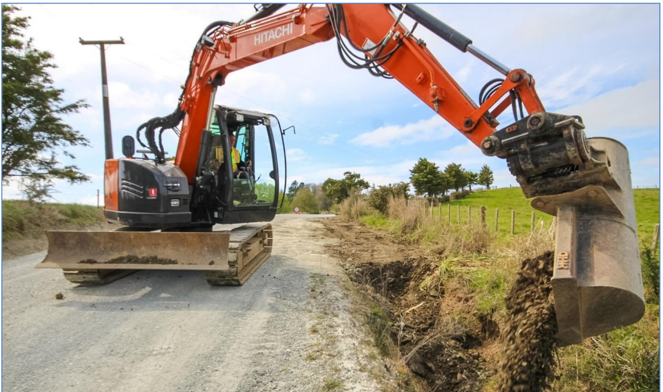
Roadside Table Drain Repair - Knight Road
