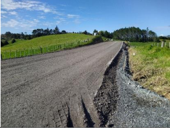
CON17086 Rd Mtce & Renewal Sth – Snooks Rd Rehab
