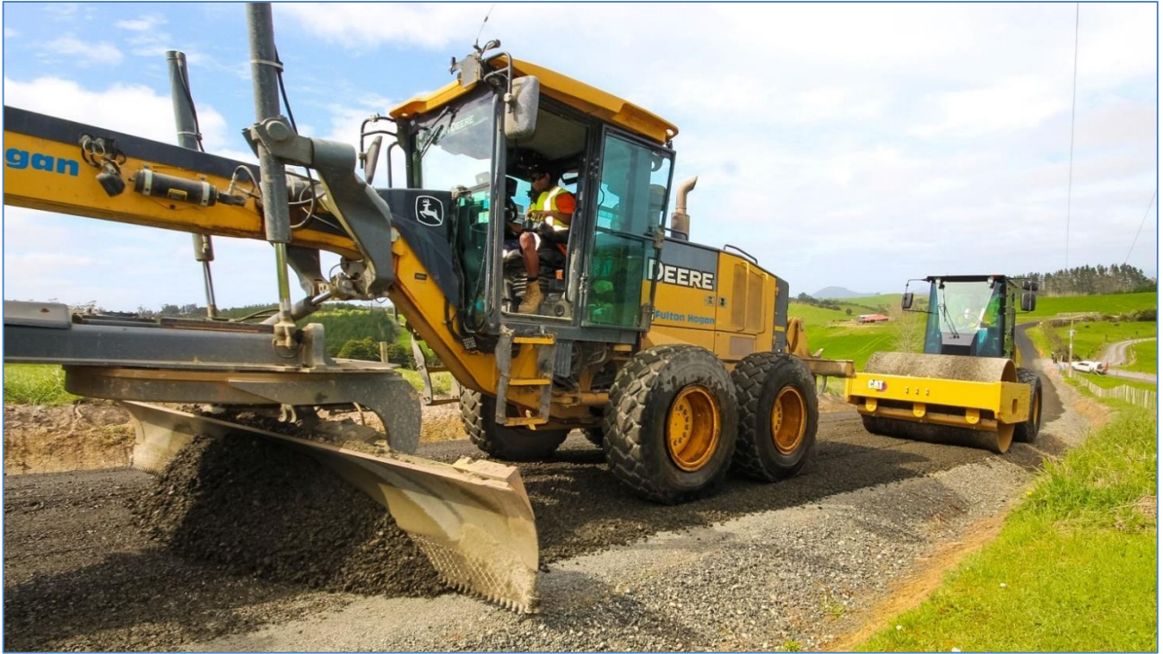
Unsealed Road Rehab - Knight Road
