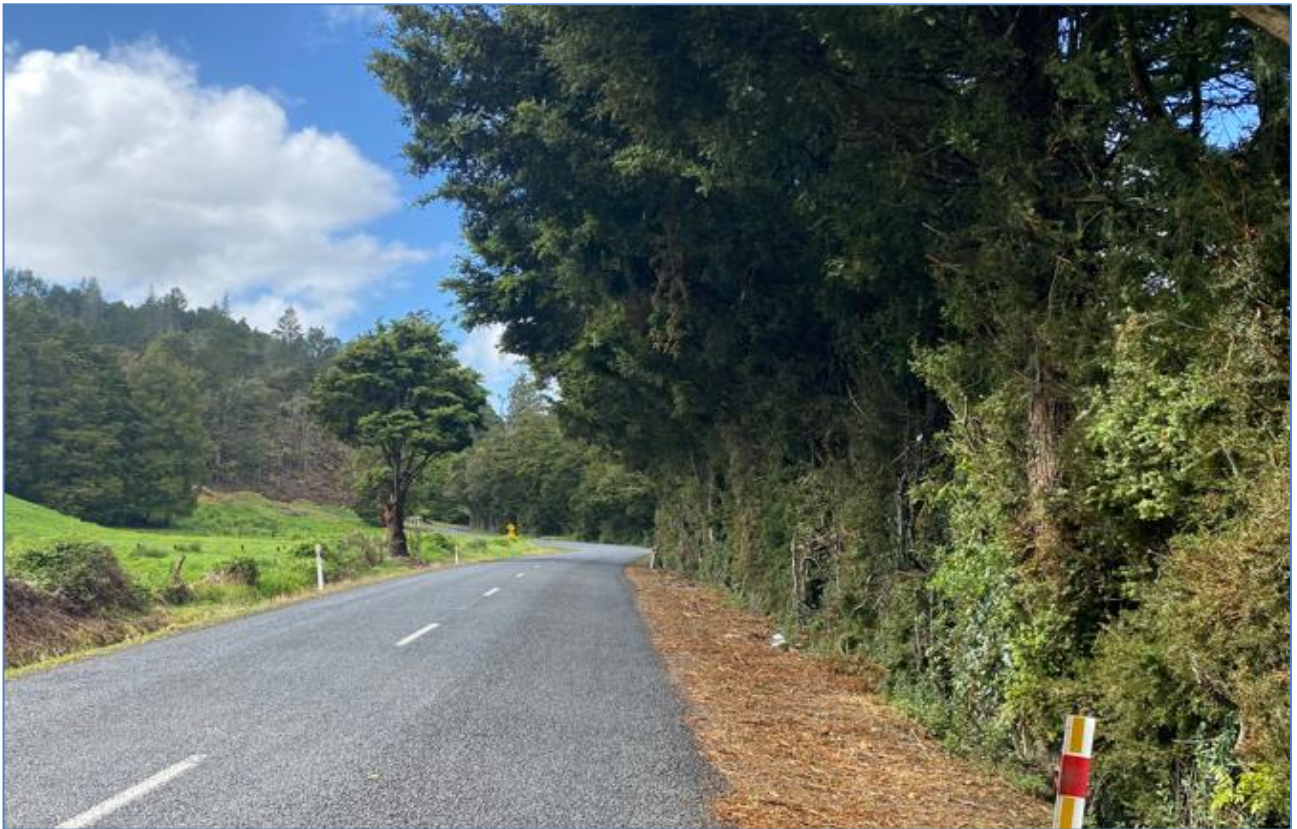
Reestablishment of vegetation envelope height – Kara Rd
