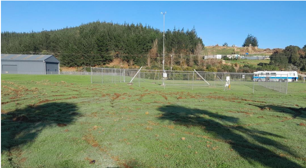
Wastewater treatment plant field damage
