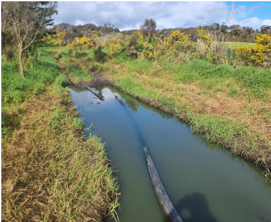
Four Wheel Vehicle Driven over track / pond at Ruakaka severing pipe
