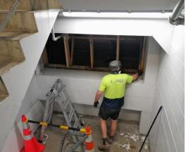
The old shingle canopy roof of the Central City Car Park has been replaced with new iron. Rot has been removed from the stairwell and some painting undertaken.
