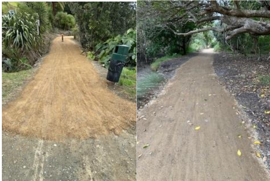
Agregate Replacement Waimahanga Track
