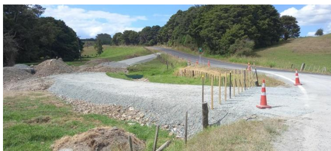
CON22086: Aponga, White and Paparoa Road Culvert Replacement – Construction of temporary crossing at Paparoa.
