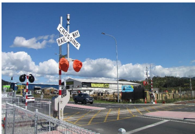
CON21015 Port Kioreroa Roundabout – Signals and barrier arms at Kioreroa Rd rail crossing
