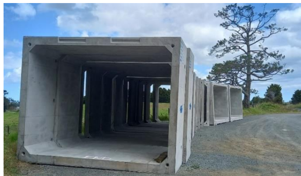
CON22086: Aponga, White and Paparoa Road Culvert Replacement – Stored culvert units for Paparoa.
