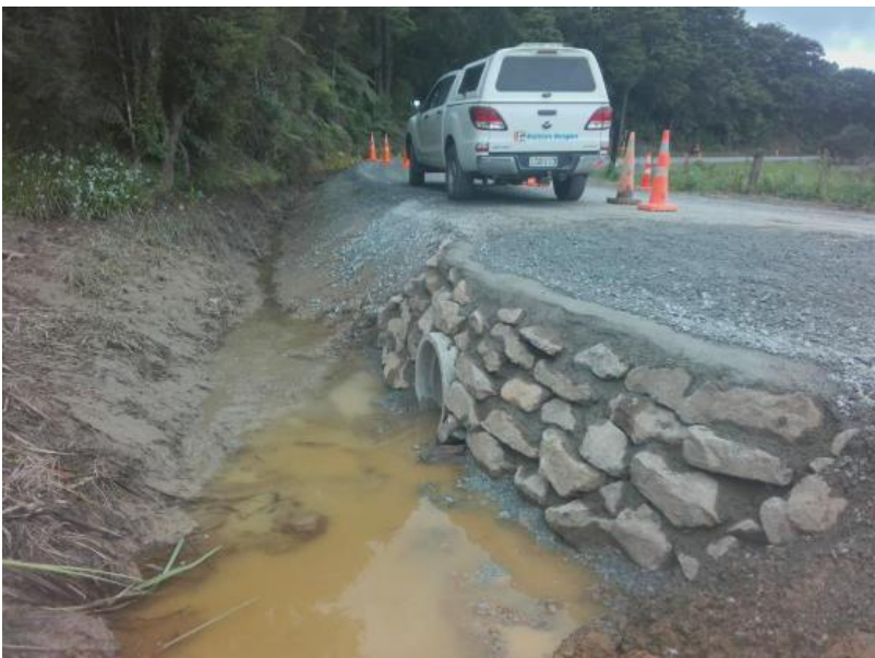
Completed head wall structure and culvert replacement on Whananaki South Road
