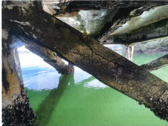
Figure 5 - RC Brace (Cracked)
