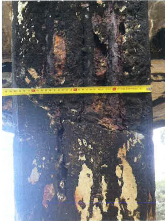
Figure 3 - RC Pile (Concrete Loss & Reinforcement Corrosion)
