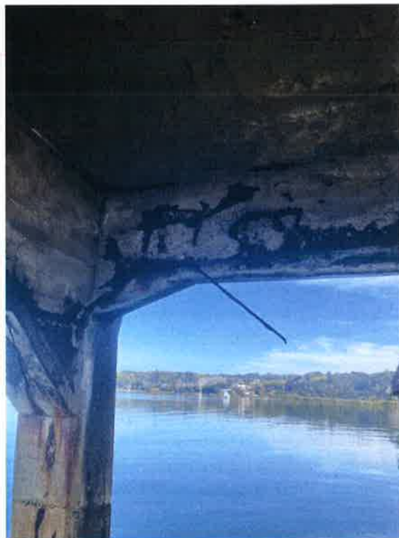
Figure 4 - RC Transverse Beam (Reinforcement Failure)
