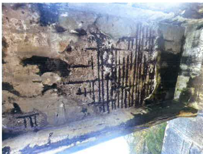
Figure 1 - Underside of RC Deck (Adjacent to Shore Abutment)
