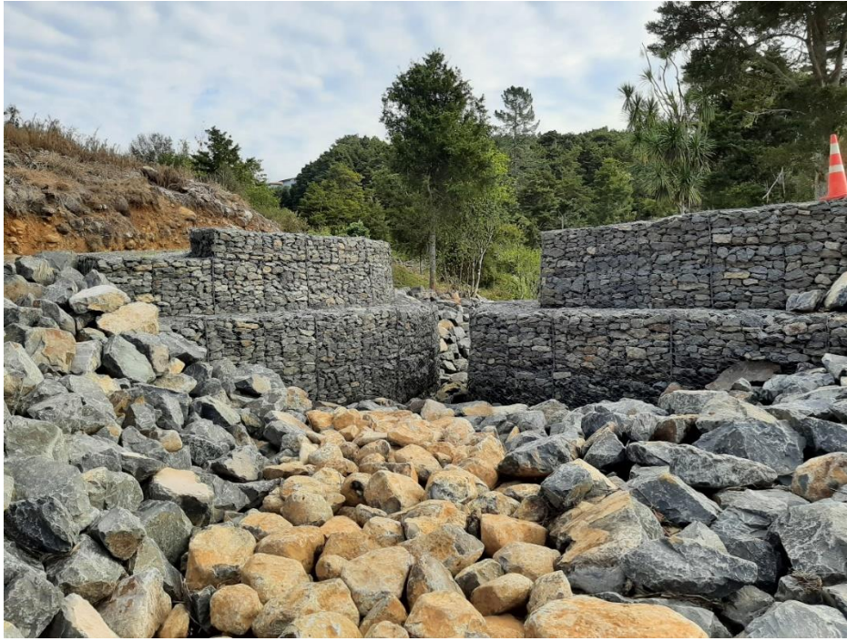
Gabion weir at the Sands Road development
