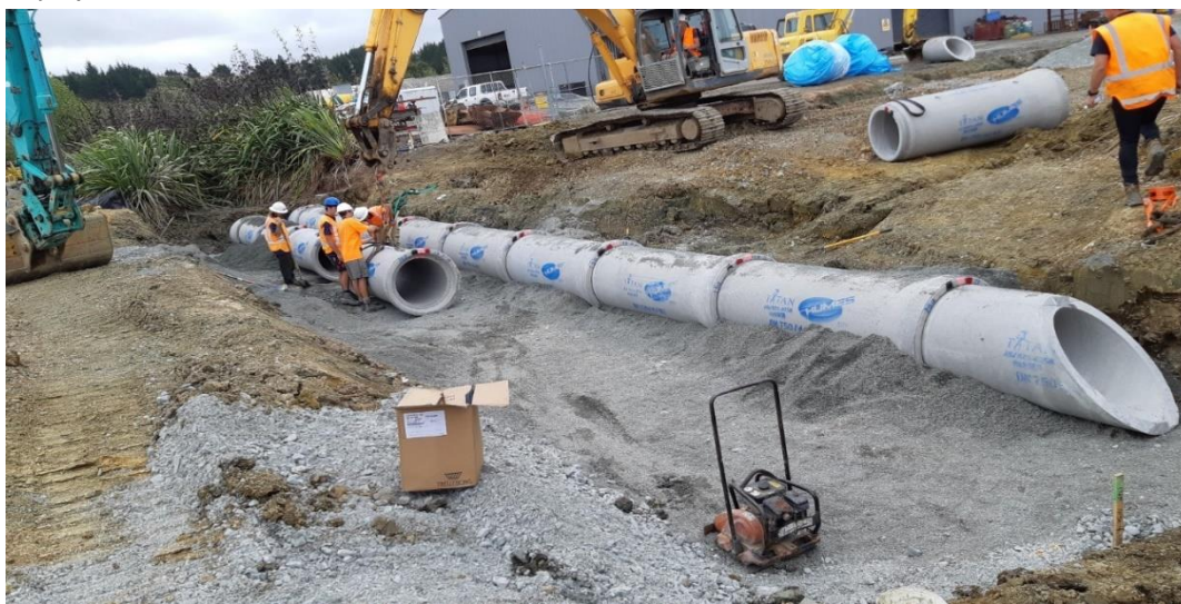
Culvert installation at Logyard Road
