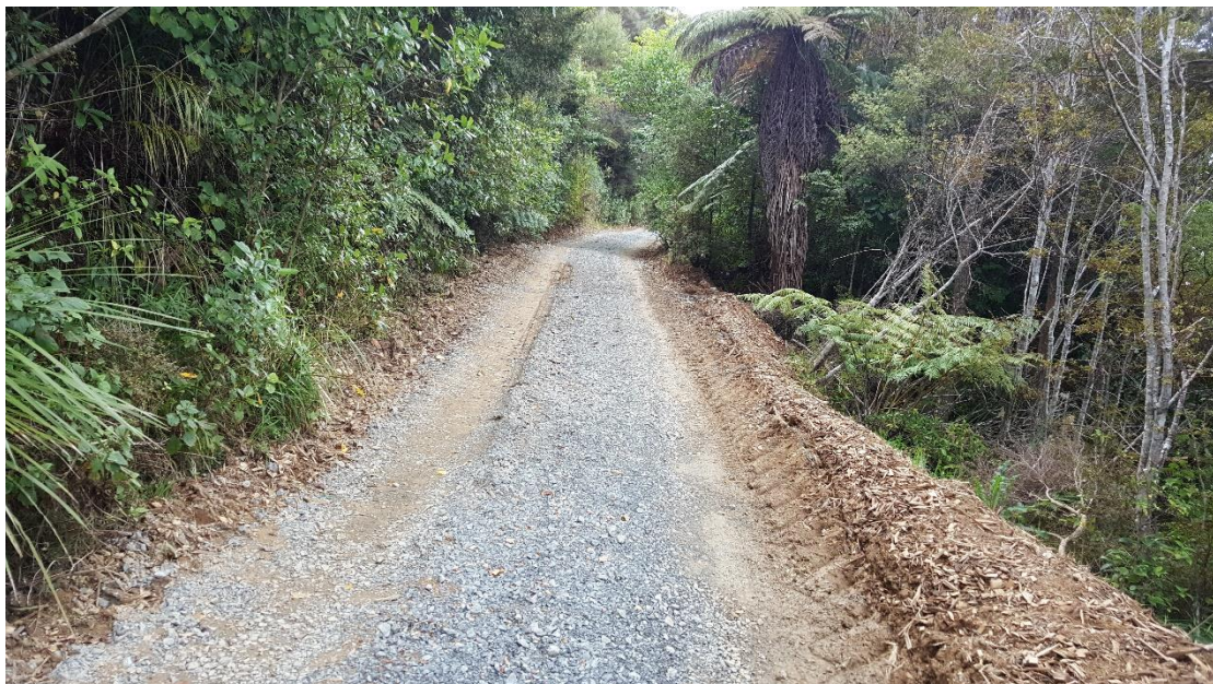
Example of the upgraded track
