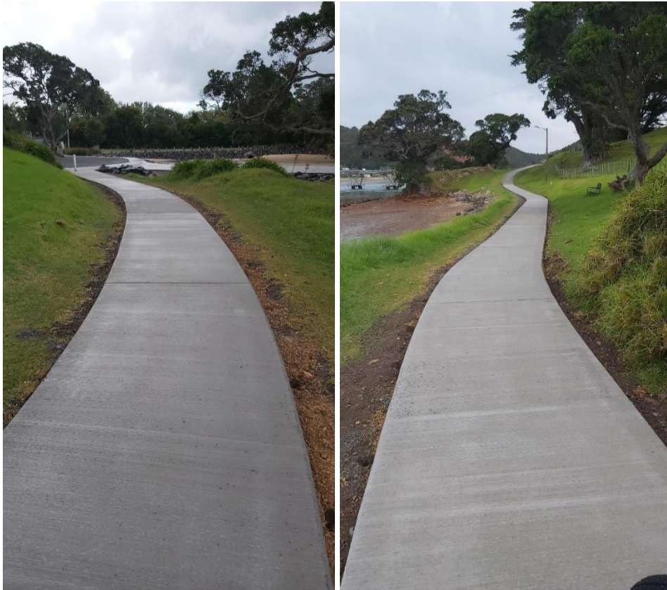
Pataua North completed walkway section
