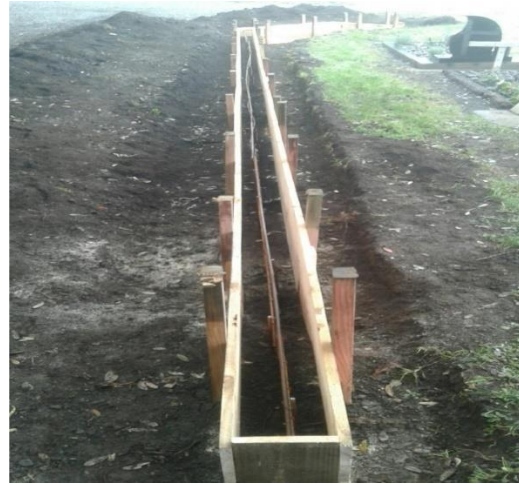
Nib wall under construction to prevent further damage
