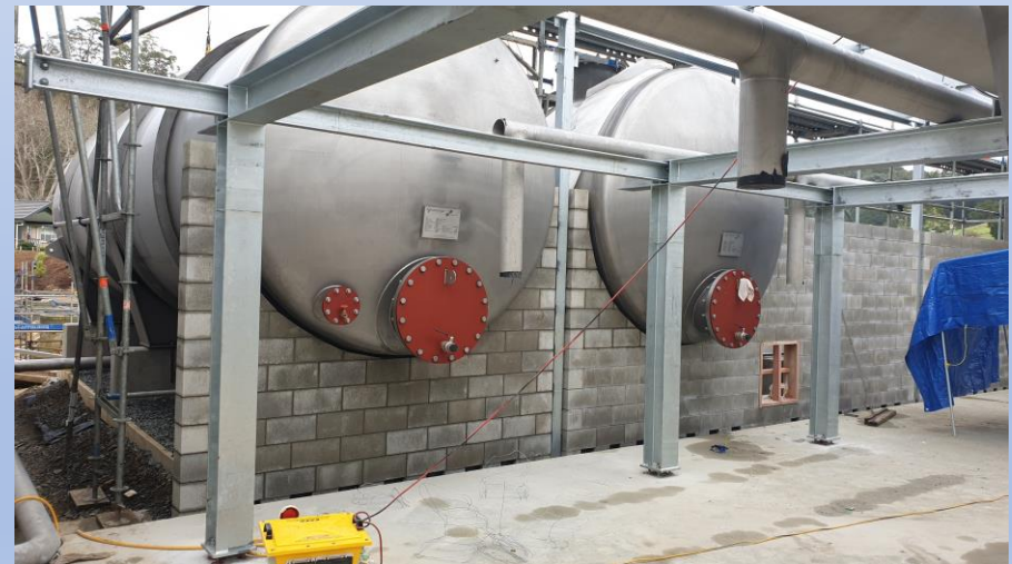
BAC Filters installed
