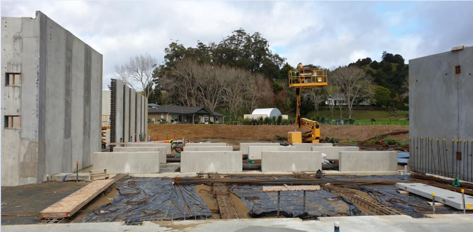
Foundations for BAC Filters
