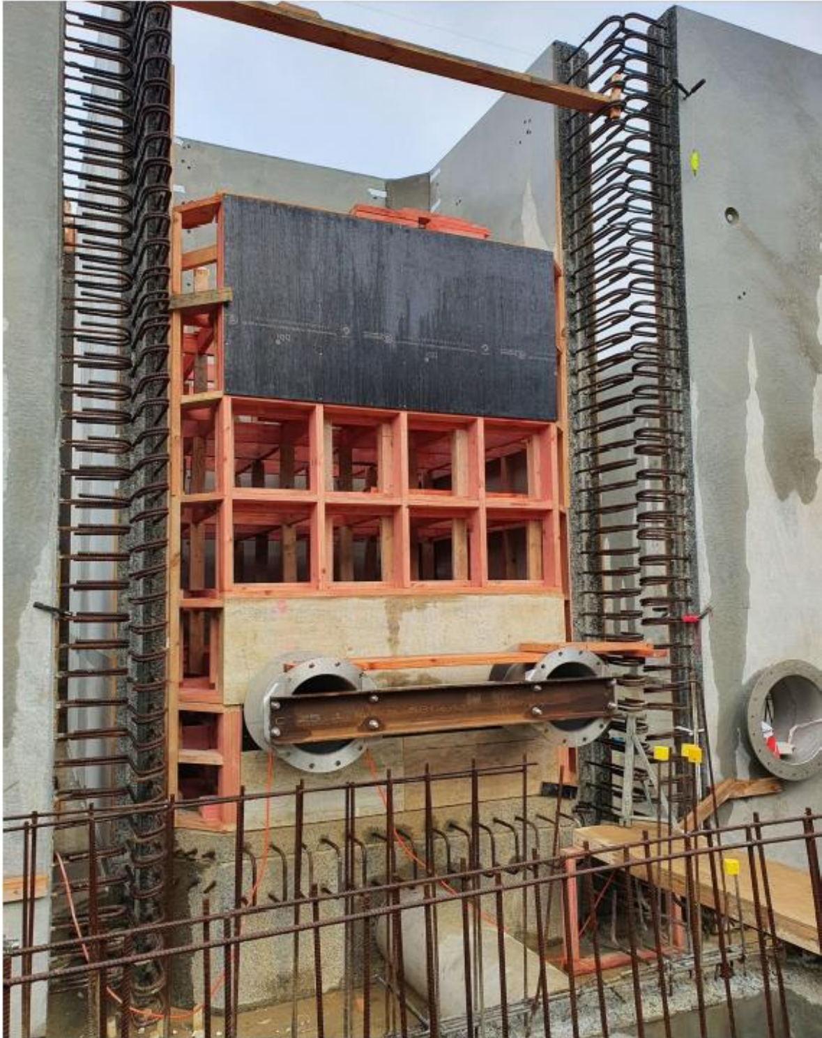
Figure 3 - Stich joint between pre-cast panels May 2020
