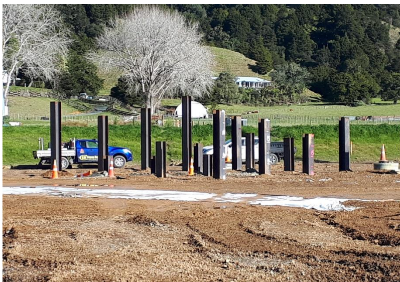
Piling operations underway at the new water treatment plant site – Whau Valley
