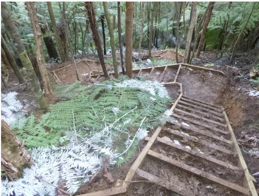
Mackesy Bush walking track upgrade. New Steps awaiting surfacing.
