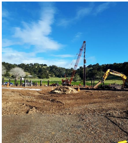
Piling operations underway at the new water treatment plant site – Whau Valley
