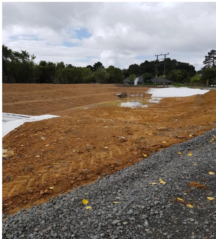
Stormwater treatment Pond at the New Whau Valley WTP
