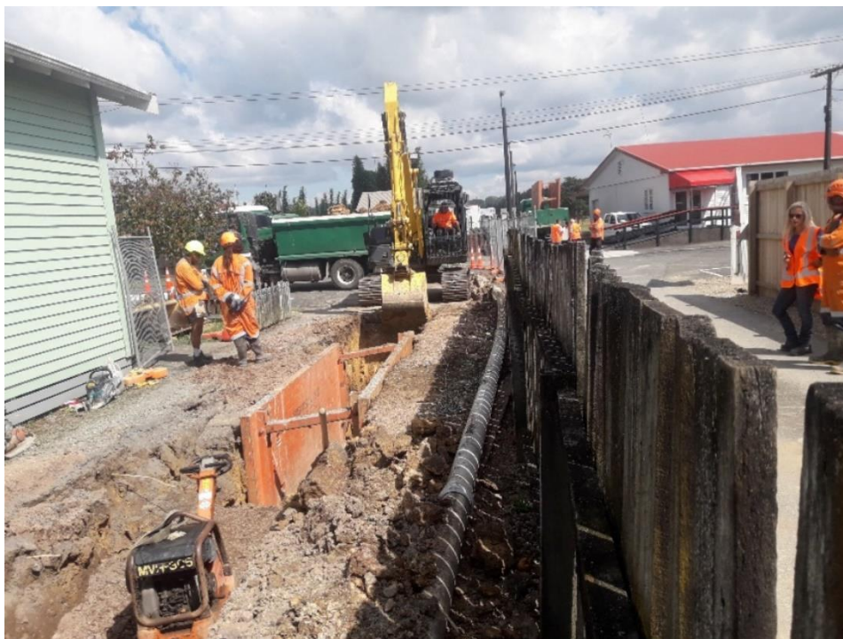
Gravity Sewer Upgrade at Park St, Hikurangi
