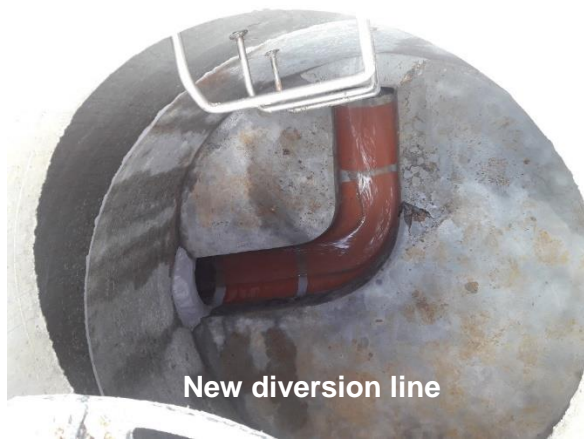
New 300mm line diversion manhole at Takahe St now in operation
