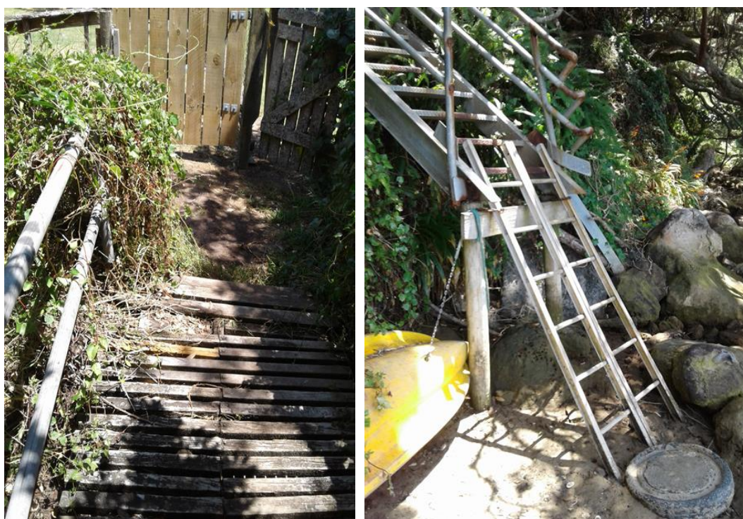
76-84 Marsden Point Rd - non-complying steel steps
