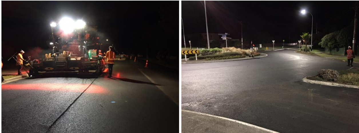
Kiripaka Rd resurfacing operations
